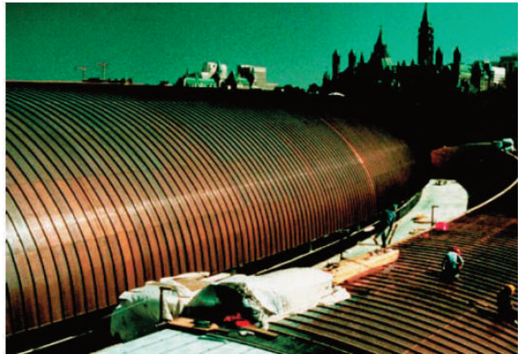
Batten seam copper roof, Museum of Civilization, Hull.
