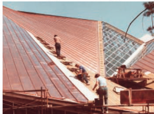
The bright salmon colour of bare copper (left at the Metro Toronto Zoo) will evolve, in Eastern Canada and on the West Coast, into the familiar grey/green patina (above).
