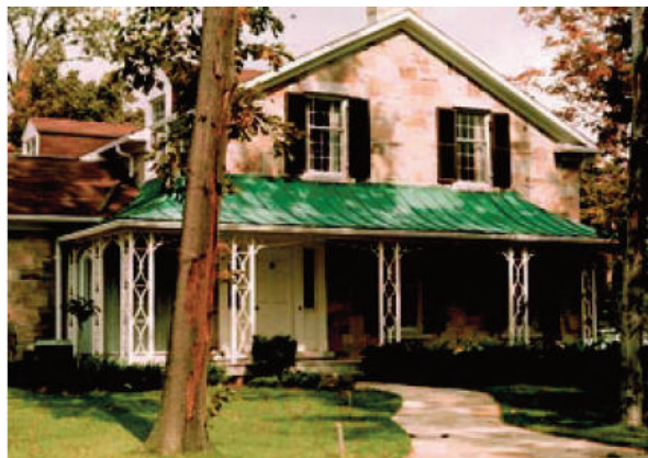
Above: Prepatinated copper standing seam roof, Thompson House, Blenheim, Ontario.
